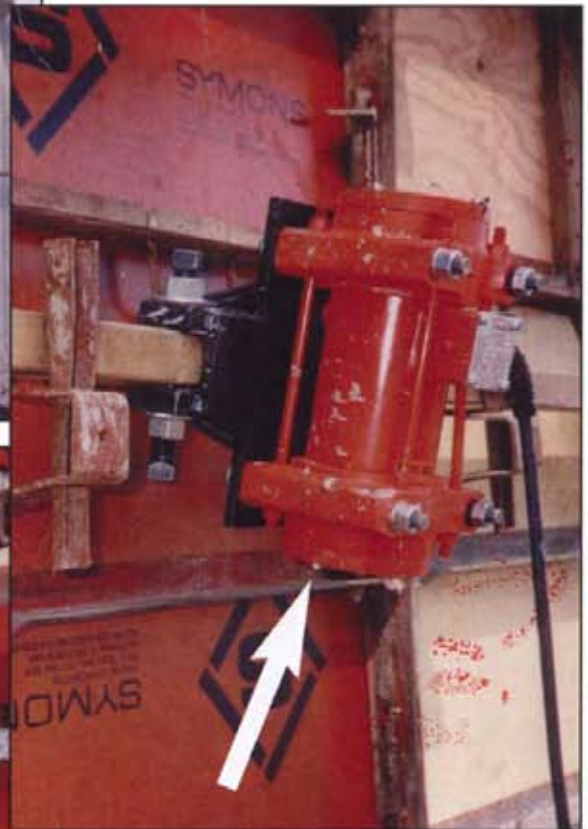
Bracket with vibrator clamped to a 2 x 6.
